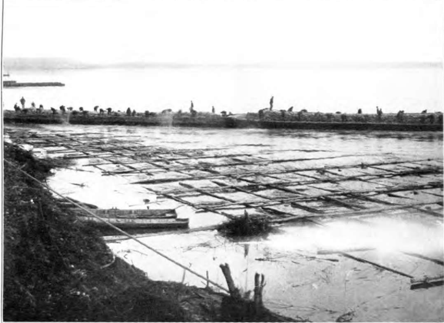
NO. 7.—SINKING SUBAQUEOUS MAT—CLOSE OF THE OPERATION.
